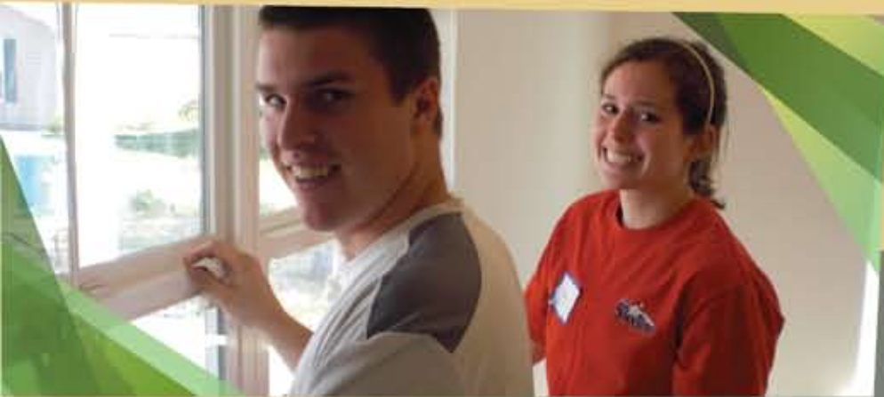
Furman students do a final window check on a Habitat home they have helped build.
